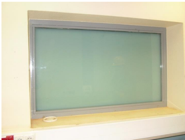
Figure 4 The clouding of fire resistant glass with a silicate gel.
