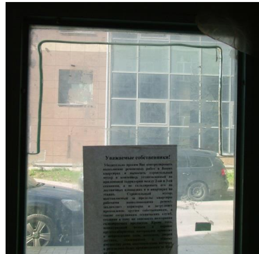
Figure 3. Syneresis in fire resistant glass with a alkali-silicate gel.
