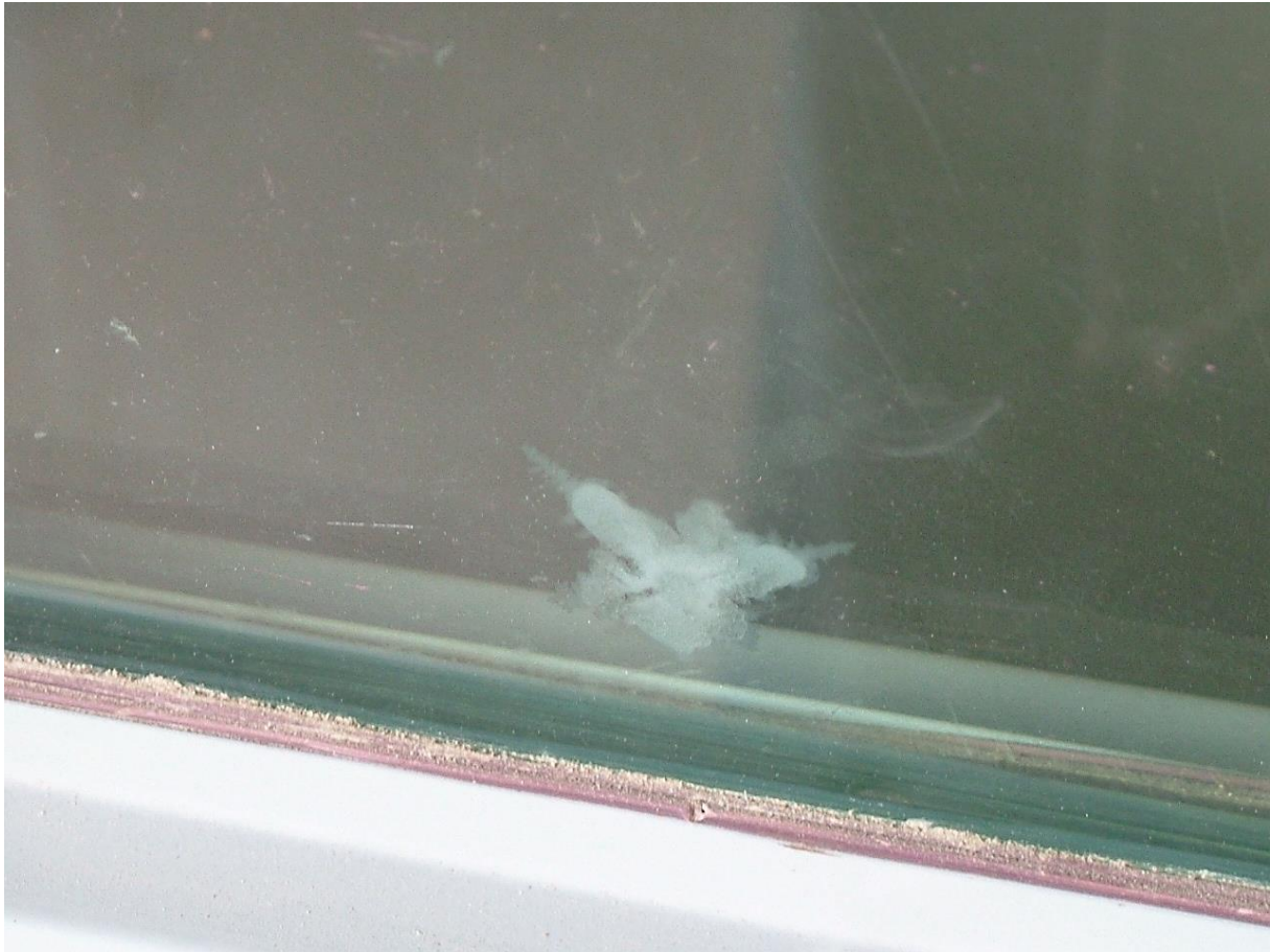
Fig 3. The aftermath of freezing of laminated glass with silicate based gel.
